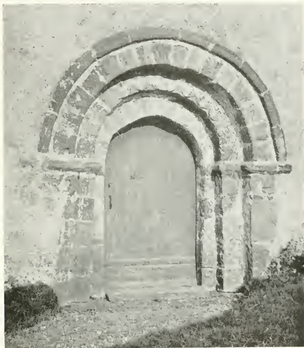
Norman Doorway, Overton Church
